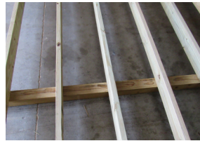
Floor Joists 12" on-center
